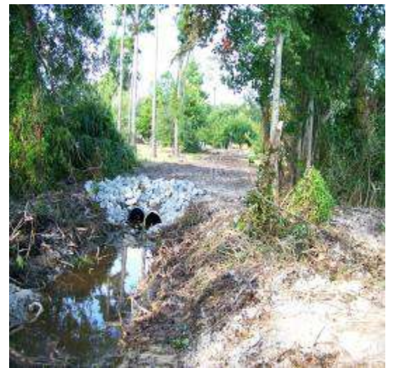
Fig. 6 New "G Outfall" to Swale
