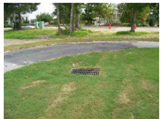
Fig. 2, new inlet & drain at cart path
