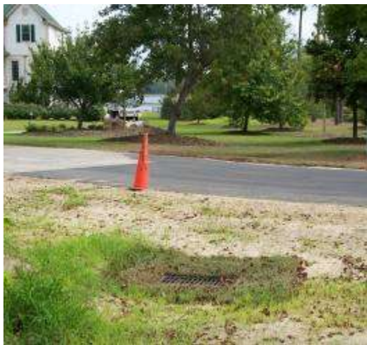
Figure 7, Completed "west j-box" & lot 315
