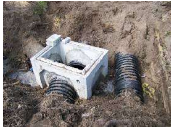
Fig. 5, tie in of existing drain
