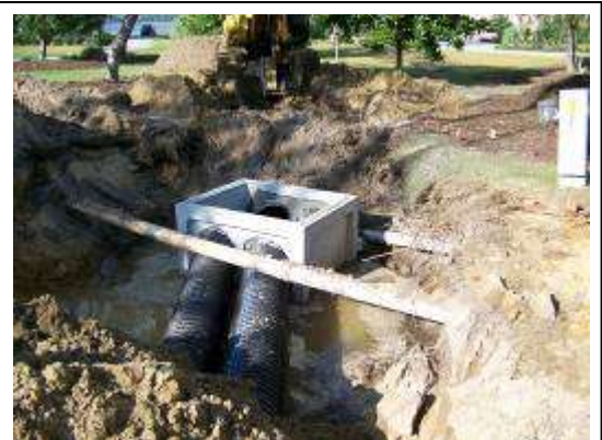
Fig. 3, East J-box connections
